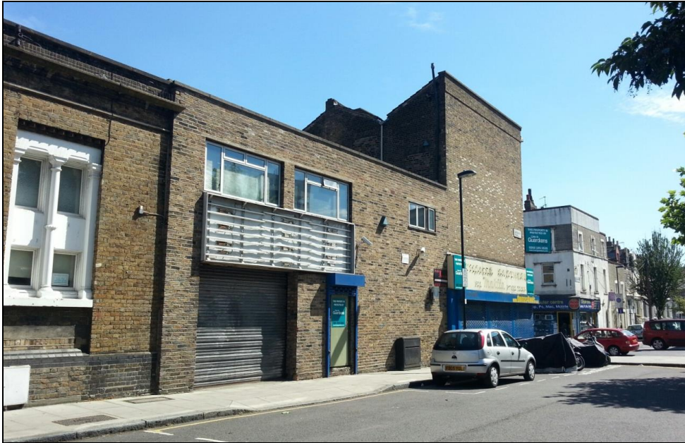
Image 3: Existing side elevation along Giesbach Road.
